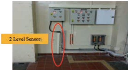
Figure 16: 2-stage Flooding Alarm
