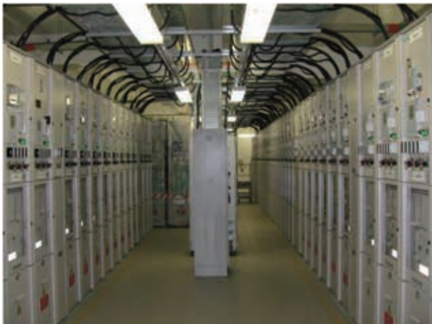
Figure 5: Lighting Design addresses Safe Operational Requirement inside Switchgear Room
