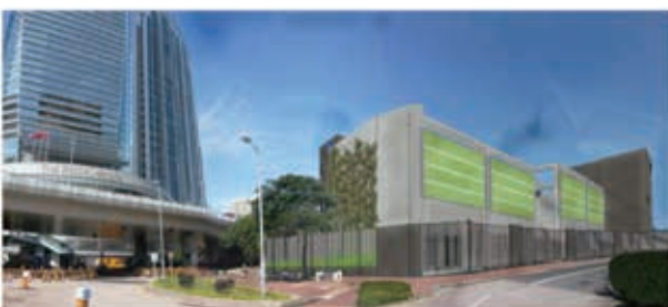
Figure 8: Substation Blends-in with Environment
