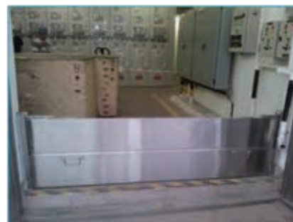
Figure 15: Installation of Flood Gate
